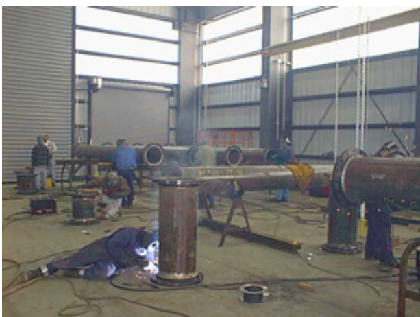
Pipe weldment in an all weather facility ensures quality.
