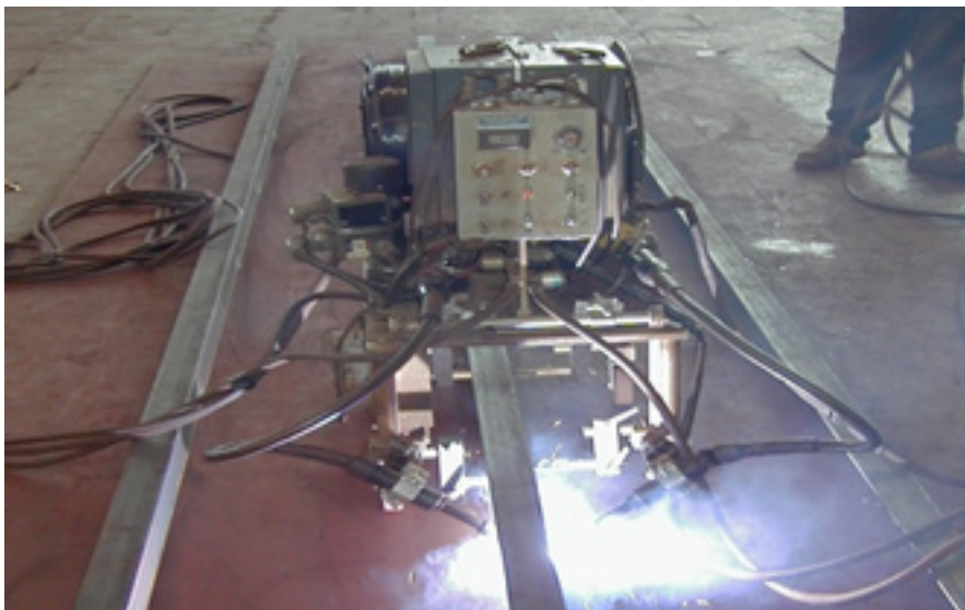
Automatic two sided structural component welder
